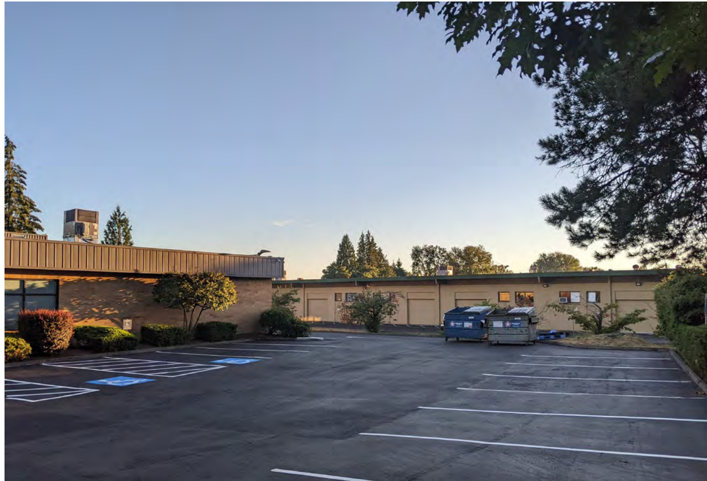
VIEW LOOKING SW - EXISTING
