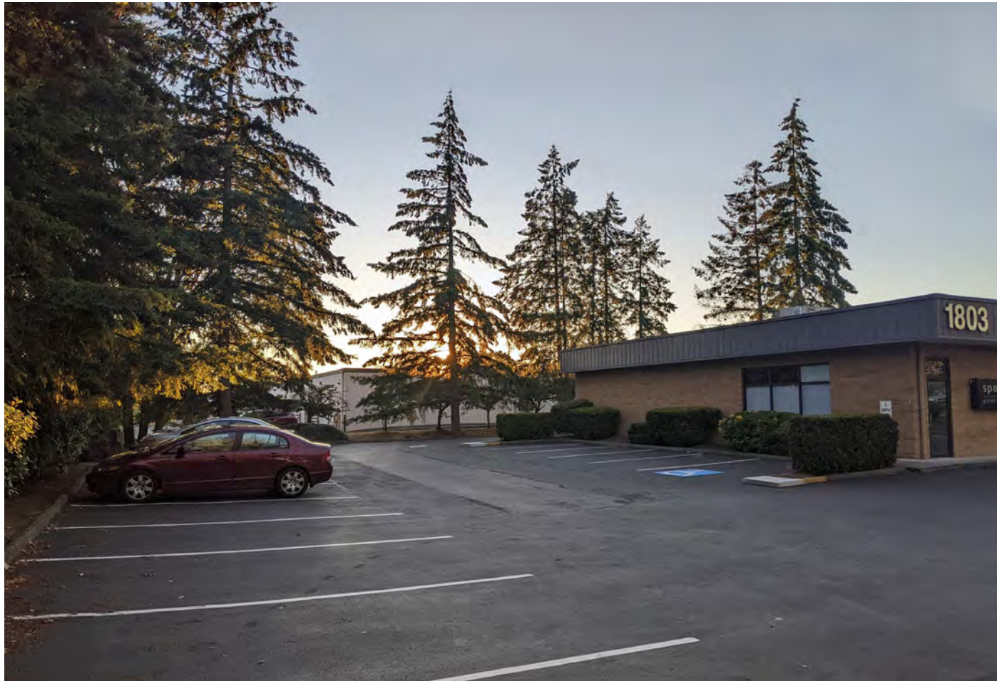
VIEW LOOKING NW - EXISTING
