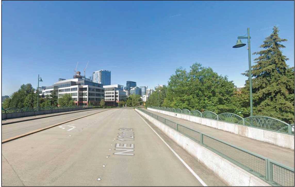
Figure 9: Existing Conditions for NE 12 th Street Over I-405 (facing west)
