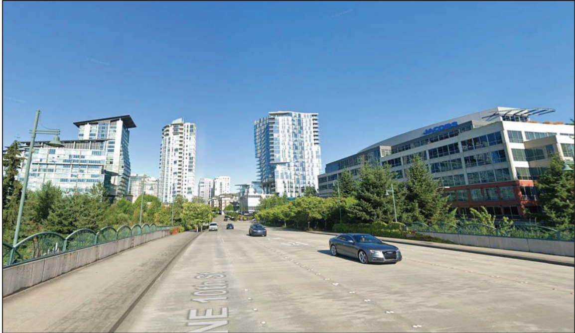
Figure 11: Existing Conditions for NE 10 th Street Over I-405 (facing west)
