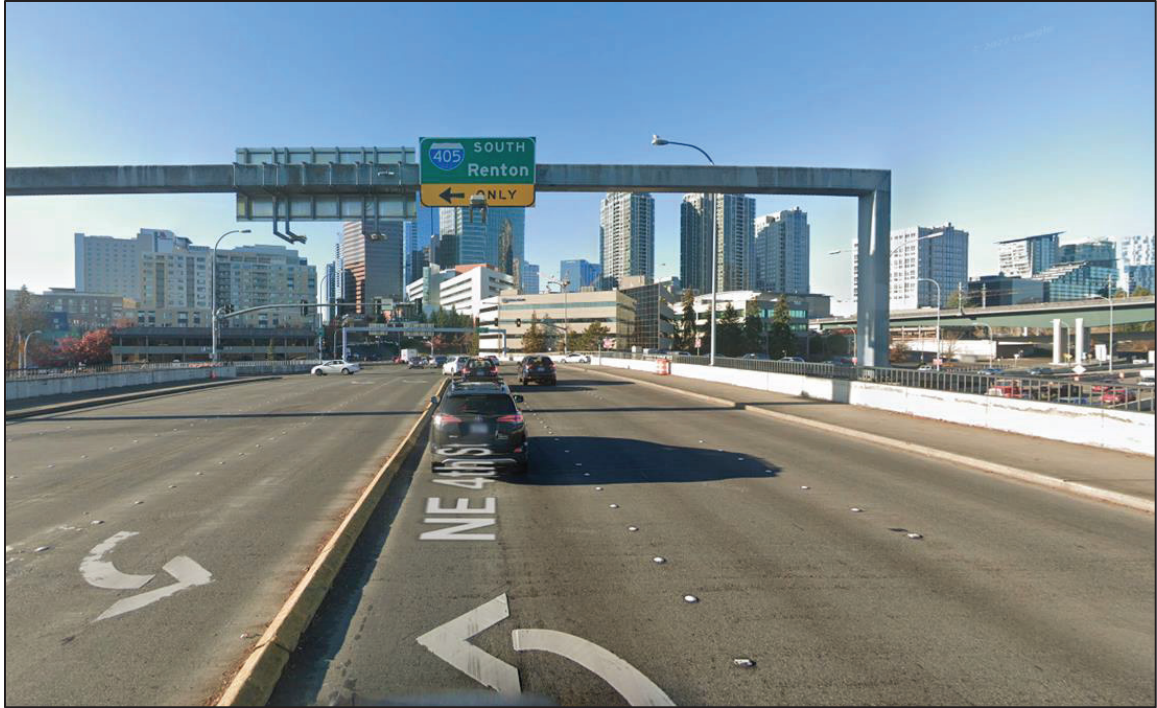
Figure 15: Existing Conditions for NE 4 th Street Over I-405 (facing west)
