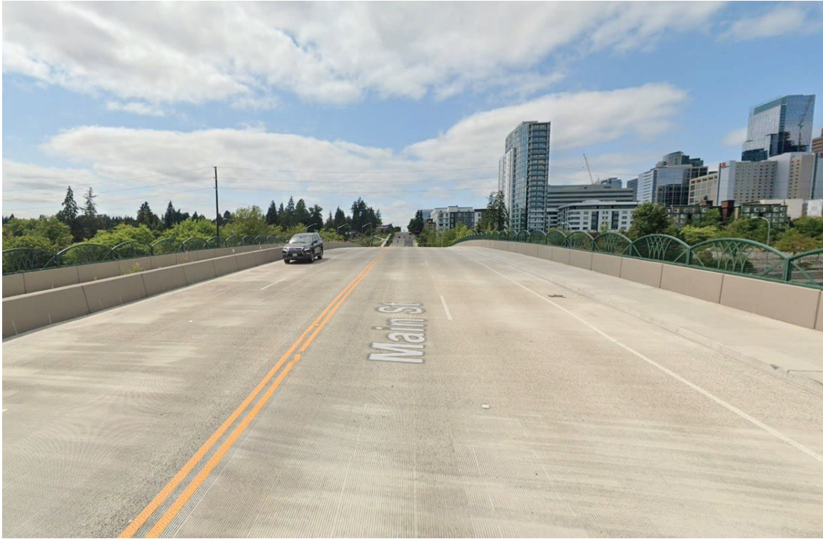
Figure 17: Existing Conditions for Main Street Over I-405 (facing west)
