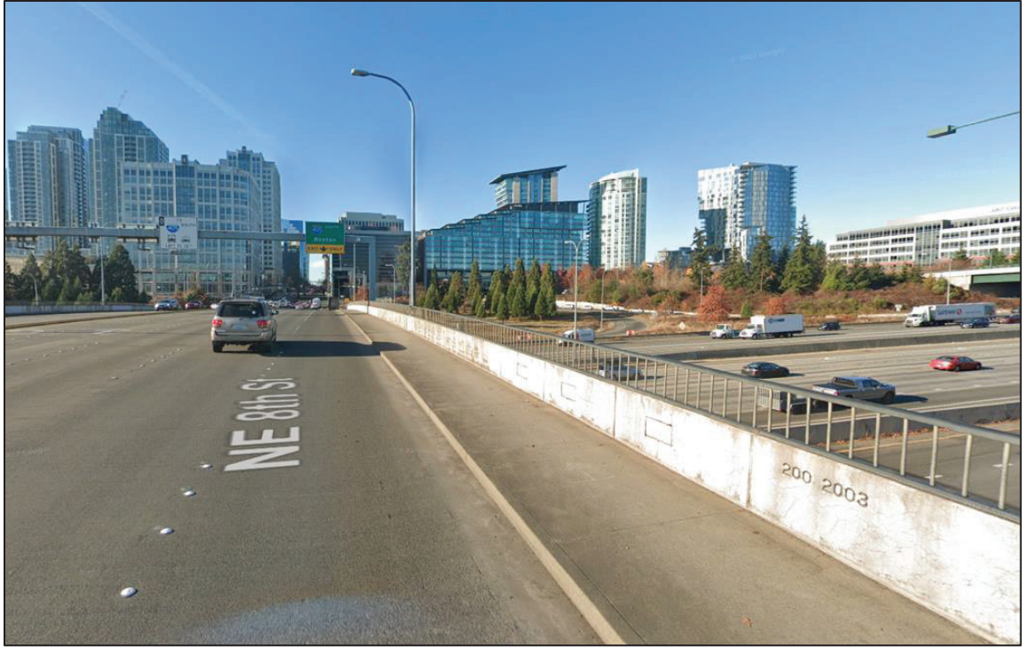
Figure 13: Existing Conditions for NE 8 th Street Over I-405 (facing west)
