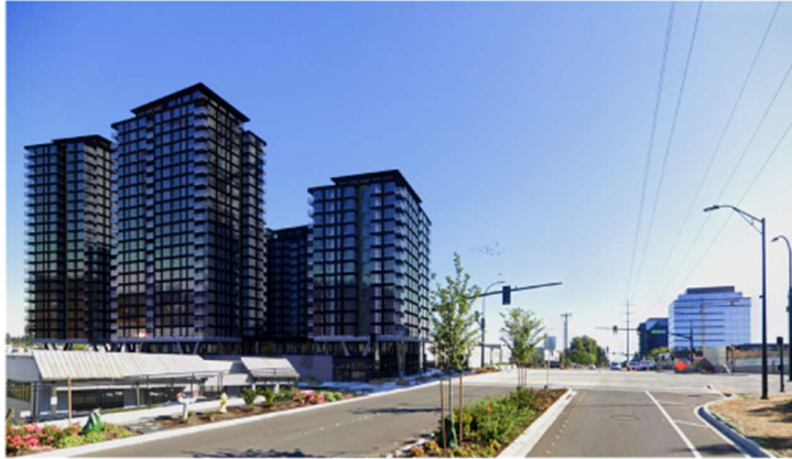
View 2 from 124th Ave NE looking south
