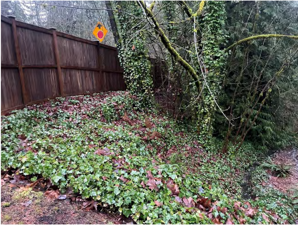
Photo 21. Location of Wall 2, standing on private drive of PN 1525059259, looking west at ditch line and backside of NE 40th Street fence. Image captured January 27, 2024, by DEA staff.
