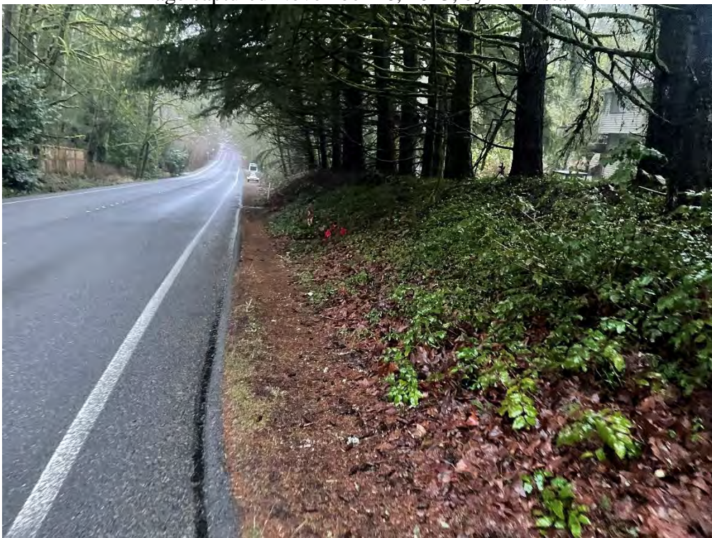
Photo 24. Location of Wall 3, standing at intersection of NE 40th street and 142nd Place NE, looking west at marked utilities and closed conveyance storm utility along north edge of NE 40th Street. Image captured January 27, 2024, by DEA staff.
