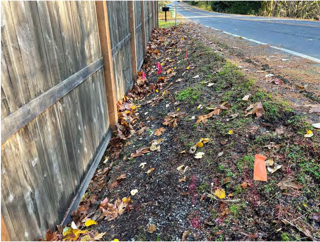
Photo 19. Location of Wall 2, standing at PN 1525059259, looking east at marked utilities and frontside of NE 40th Street fence. Image captured November 16, 2023, by DEA staff.
