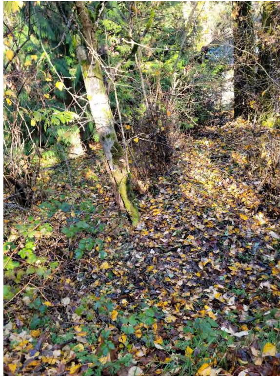
Photo 15. Ditch line at location of Wall 1 looking at DP-1. Image captured November 16, 2023, by DEA staff.
