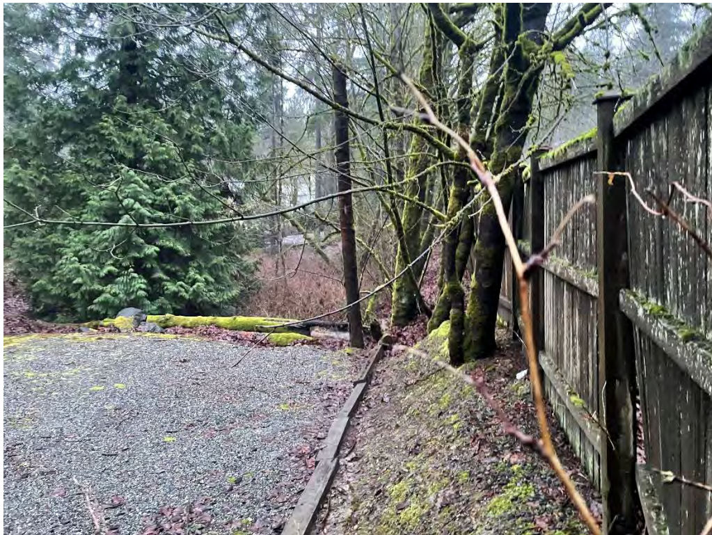
Photo 16. Location of Wall 2, standing on private driveway of PN 1525059036, looking east at backside of NE 40th Street fence toward Valley Creek. Image captured January 27, 2024, by DEA staff
