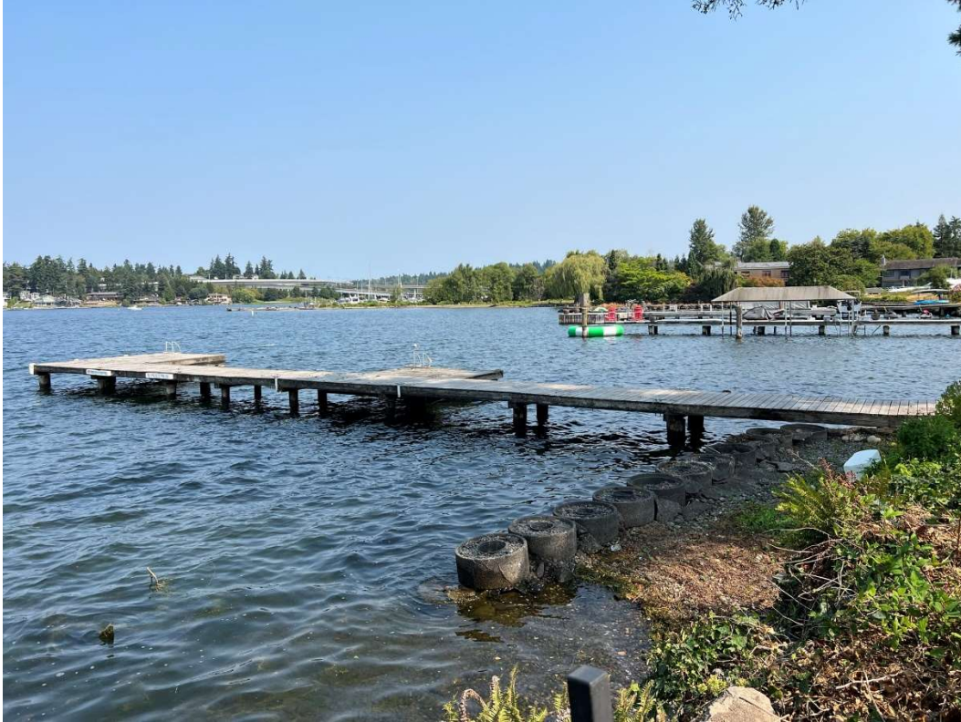
PHOTO 2 – EXISTING PEIR AND CONCRETE BREAKWATER, DATE 08/24/23
