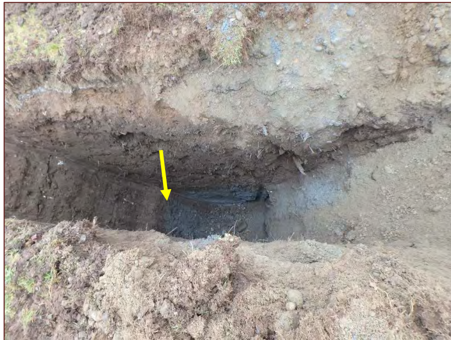
Contact Cover Soil/Landfill Debris with Native Glacial Till Soils
