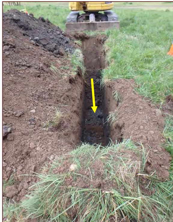
Contact Cover Soil/Landfill Debris with Native Glacial Till Soils
