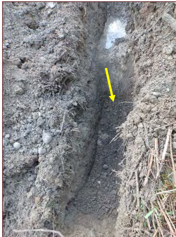
Contact with Outwash Gravel Soils
