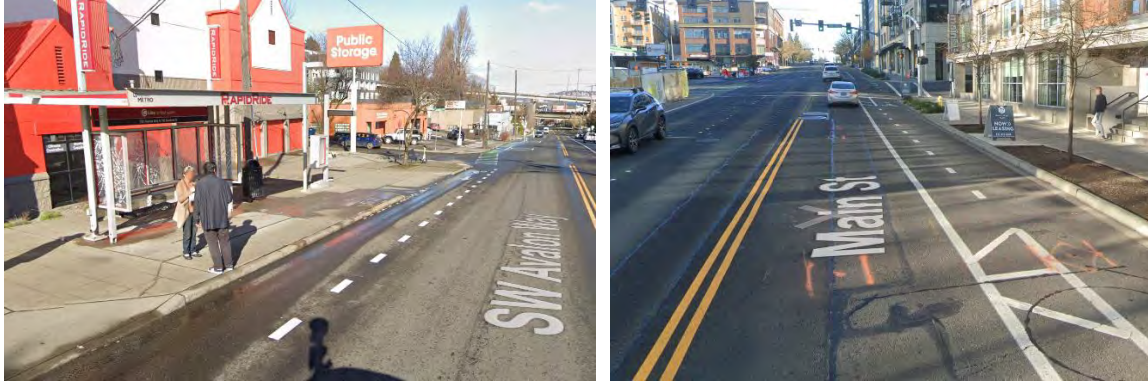
Figure 5: Skip Striping at SE Avalon Way & SW Bradford St, Seattle (Left) and at Main St & 106 th Ave, Bellevue (Right).
