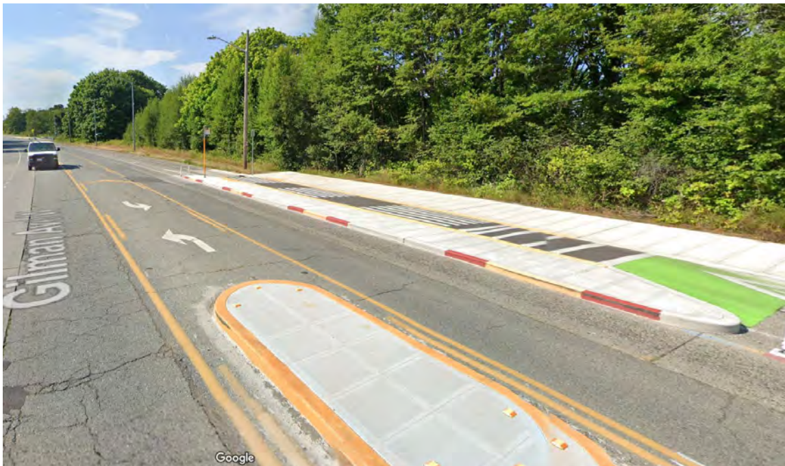
Figure 2: Island Bus Stop with Ramped Bike Lane at Gilman Ave W & 27th Ave W, Seattle, WA
