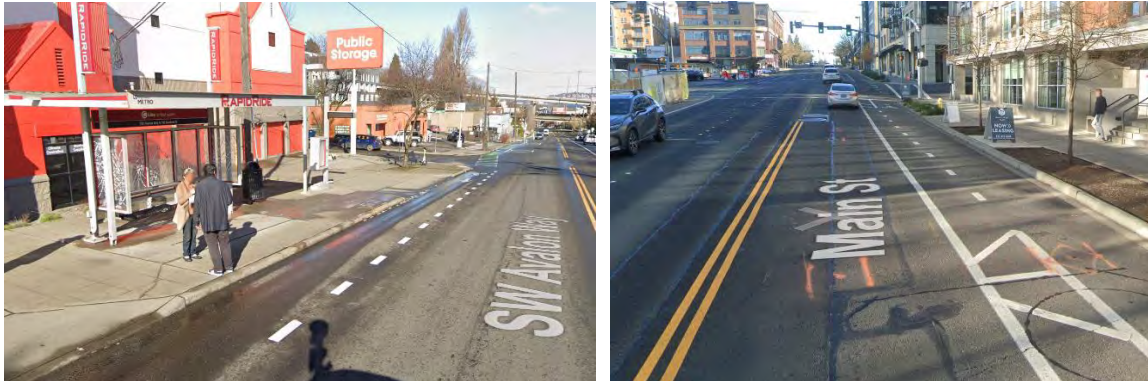
Figure 5: Skip Striping at SE Avalon Way & SW Bradford St, Seattle (Left) and at Main St & 106 th Ave, Bellevue (Right).
