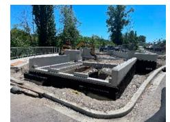
Bellevue Way SE, you will be able to see the concrete stem walls rising from the ground. The sub-grade work will be completed along with the interior slab this August.
