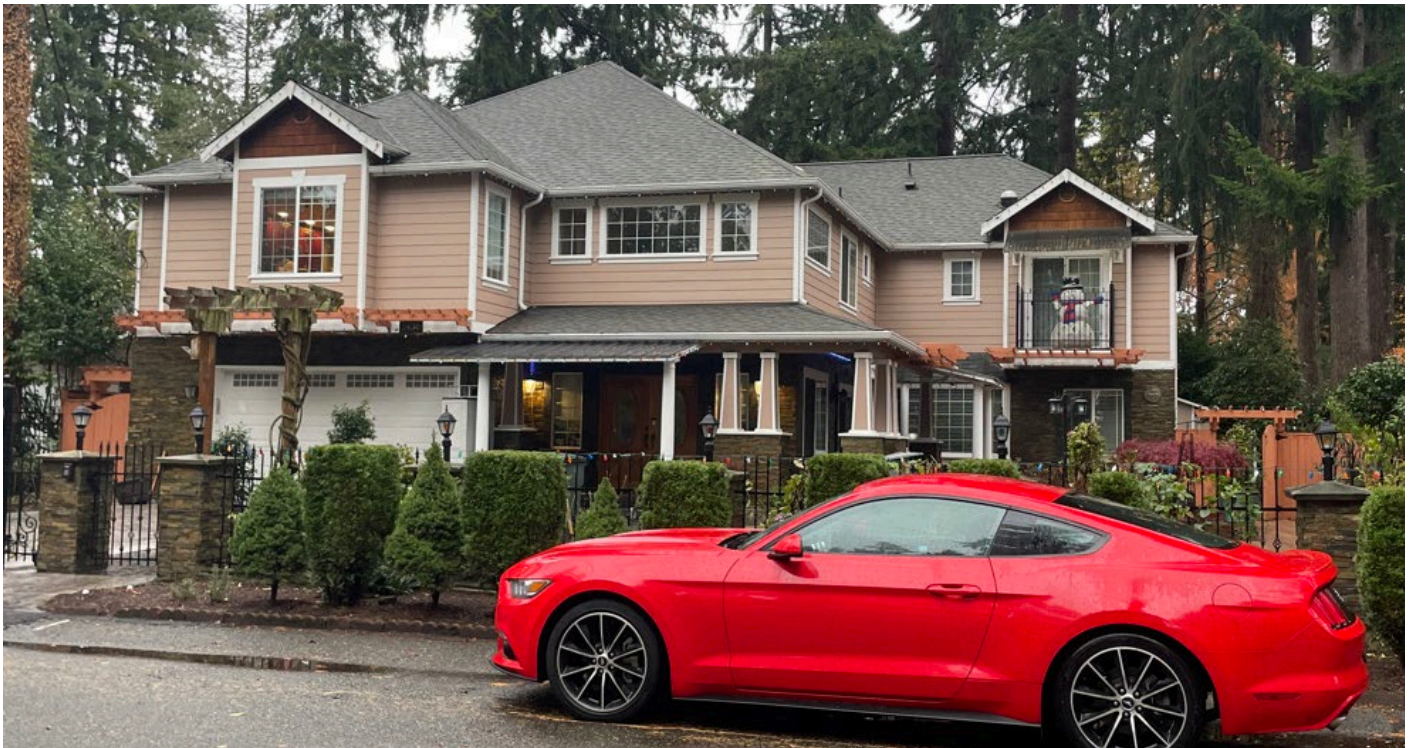
FIGURE 27 A Highly Altered Building at 2430 160th Avenue NE
