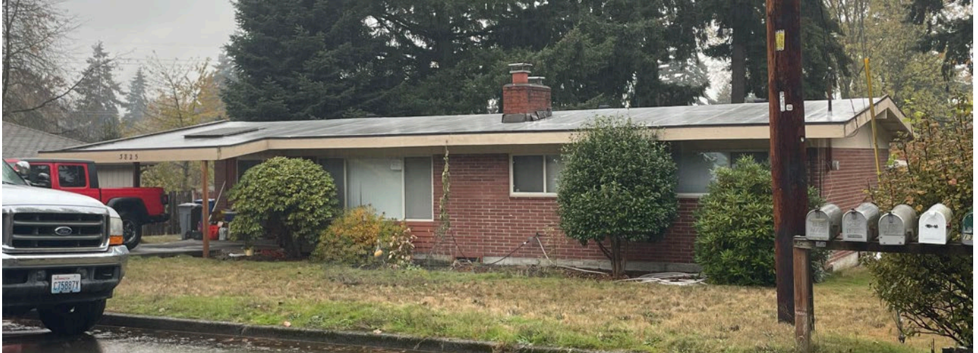
FIGURE 17 A Ranch Building at 3825 139th Avenue SE
