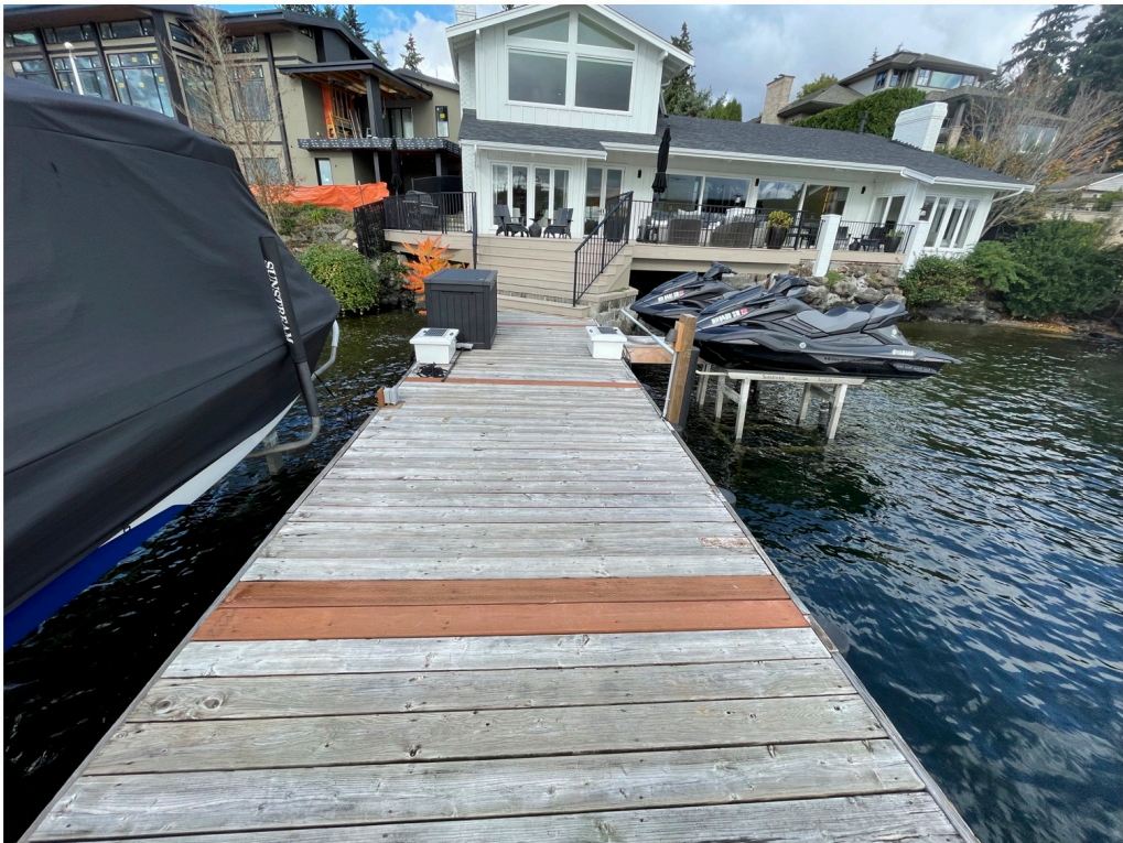
Photo 2 - Existing dock looking landward.
