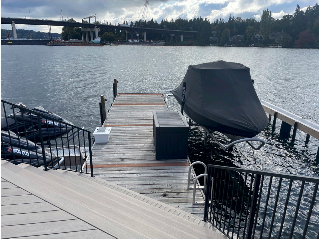
Photo 1 - Existing dock looking waterward.
