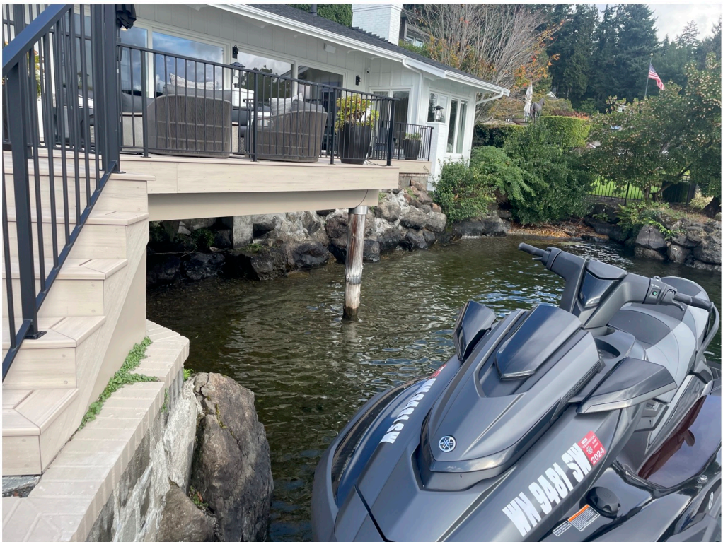
Photo 4 - Existing shoreline east of dock.
