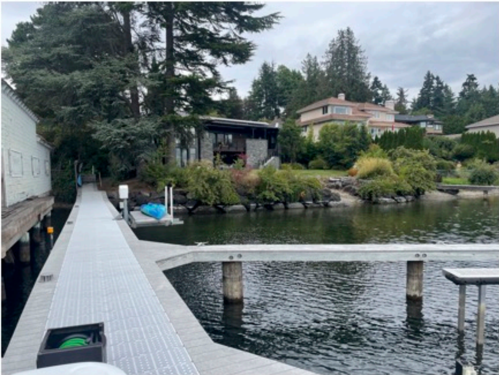
Photo 2 - Existing dock looking landward.
