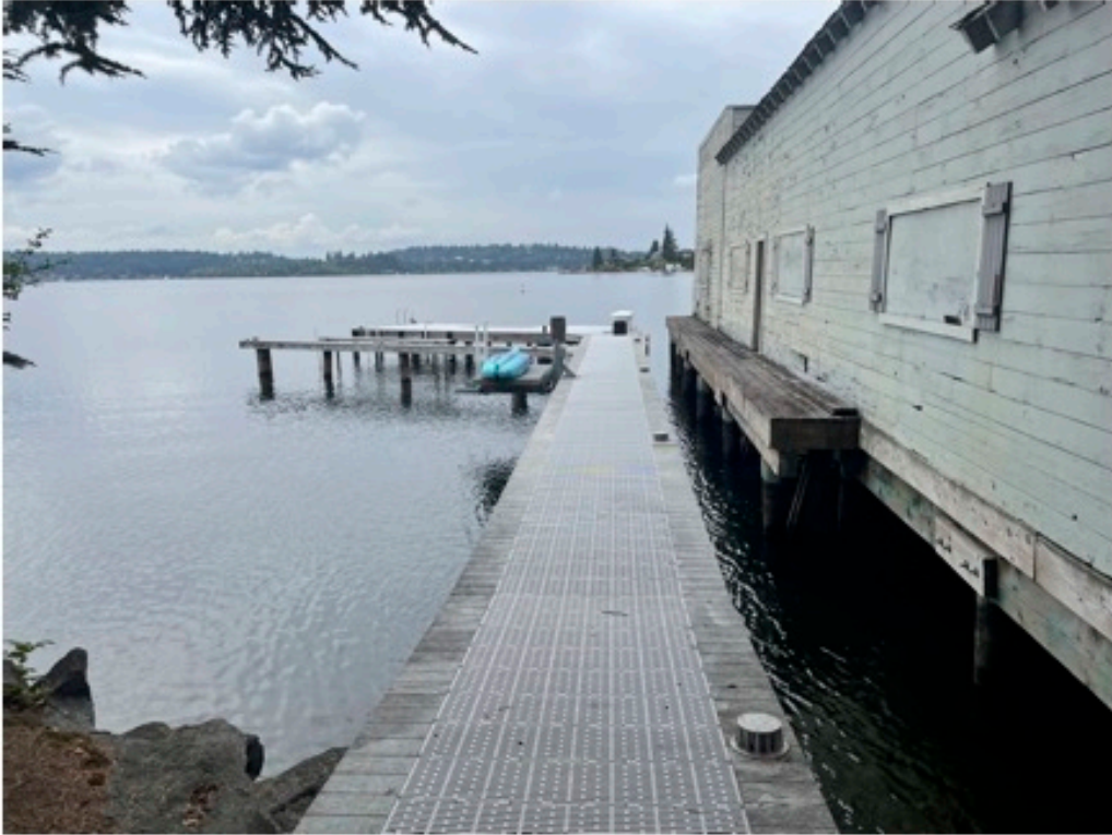
Photo 1 - Existing dock looking waterward.
