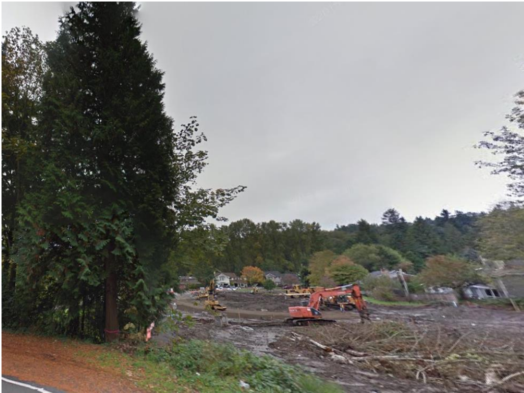
Figure 19. Google Street View image from 2015 showing clearing and grading on west side of the #31 and #32 cedars (left side of photo). Note dense, dark green canopies on the trees. There is no evidence of any tree protections present.
