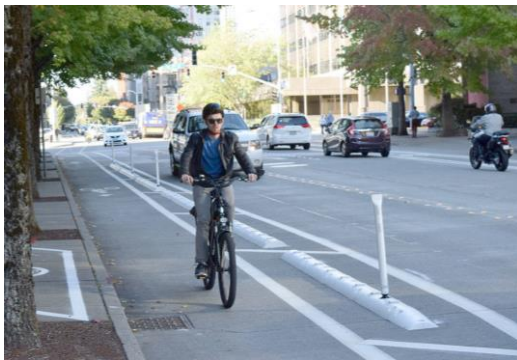
Separated Buffered Bike Lane
