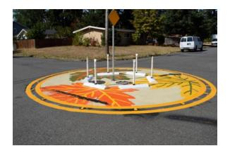
in diameter and include a decorative, thermoplastic pavement design. The circles also include interior raised, plastic curbs that were spaced at a 10-foot diameter. The center of the traffic circle contains a traffic post with yellow diamond signs for further visibility.
