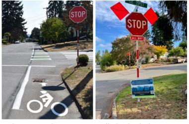
At NE 8th Street, short approach bike lanes and green markings were installed in both directions in addition to standard pedestrian crosswalk signs that were replaced with combination pedestrian plus bicyclists crossing signs to accompany the crosswalk.
