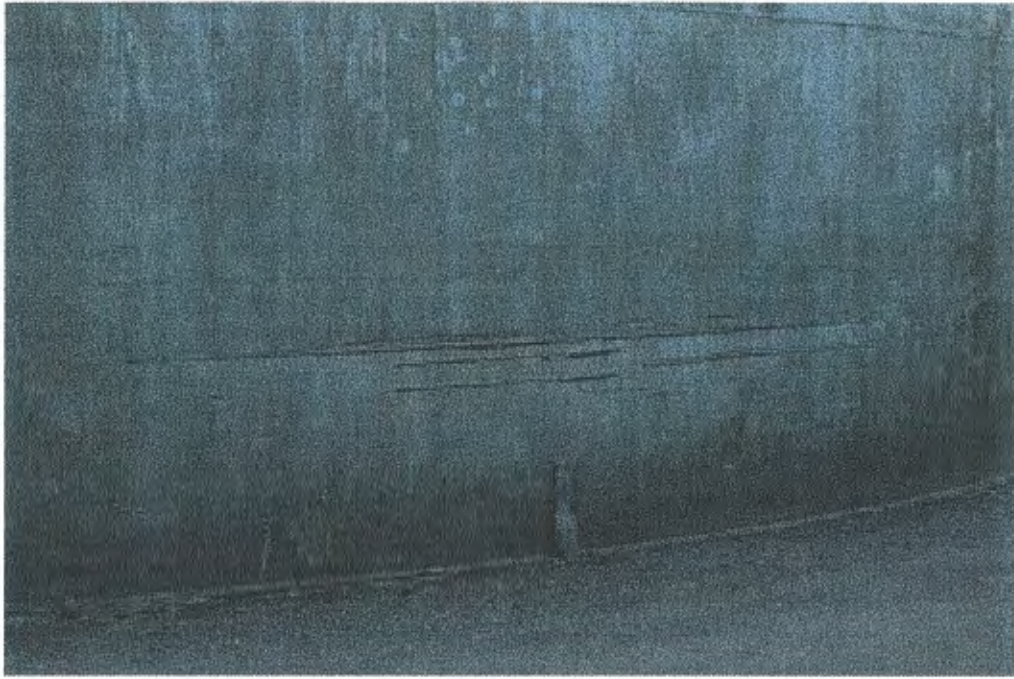
Lake Hills South - Gouged Shell Plate
