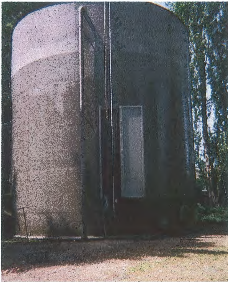
Horizon View No. 1 - Access Ladder and Overflow
