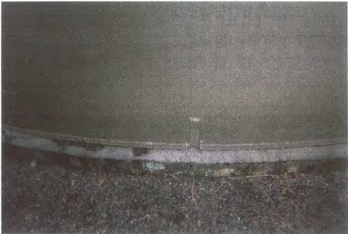
Horizon View No. 1 - Wind Anchor
