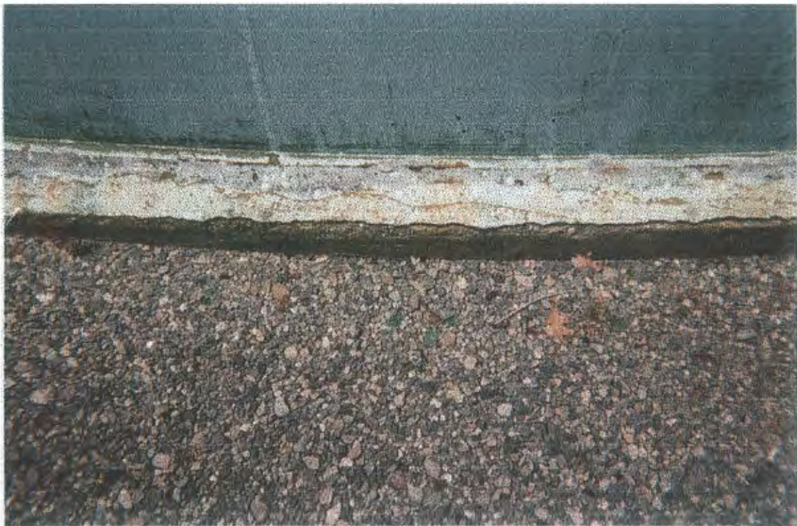
Pikes Peak - Bottom of Shell Plate at Ring Footing
