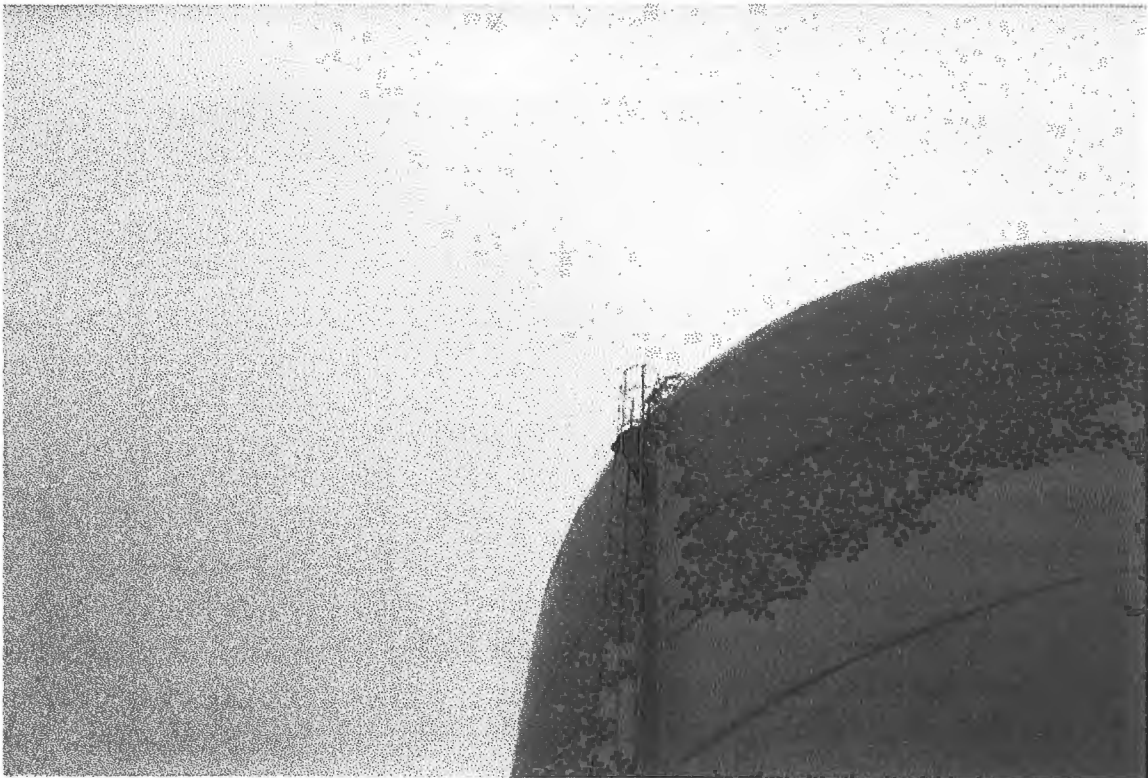
Lake Hills South - Access Ladder
