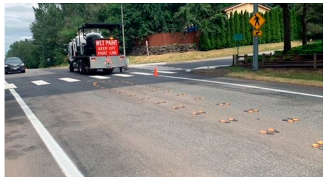
The city's contractor restriping lines along Forest Drive Southeast
