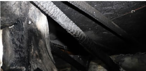
View of fire damage to the attic of the residence
