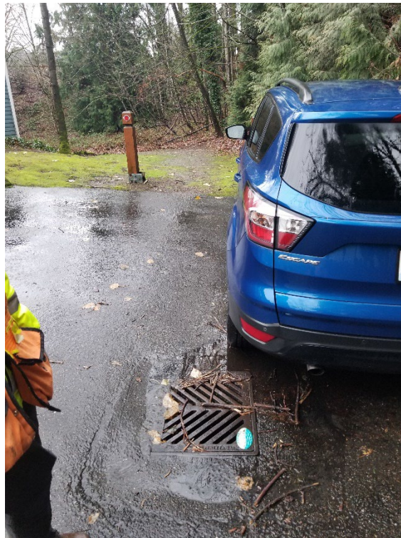
Photo 16—Second catch basin inlet to the culvert that conveys the unnamed tributary, east of TP-1 and TP-2.
