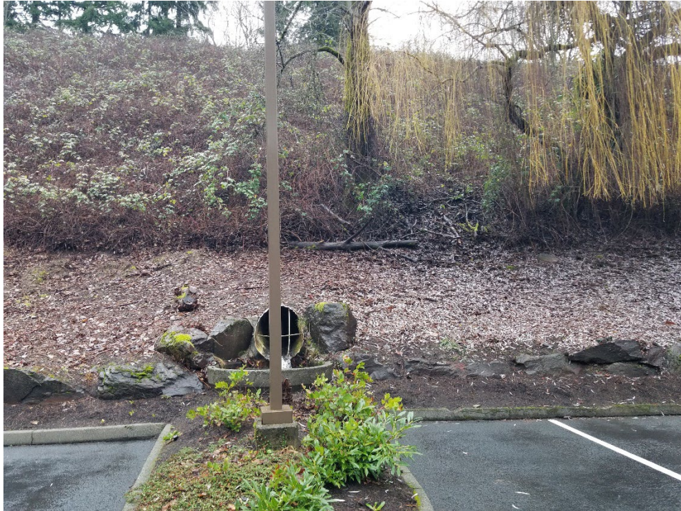
Photo 27—Unnamed tributary culvert outlet and stand pipe inlet on the SW Bel-Kirk LLC (parcel 2025059102).
