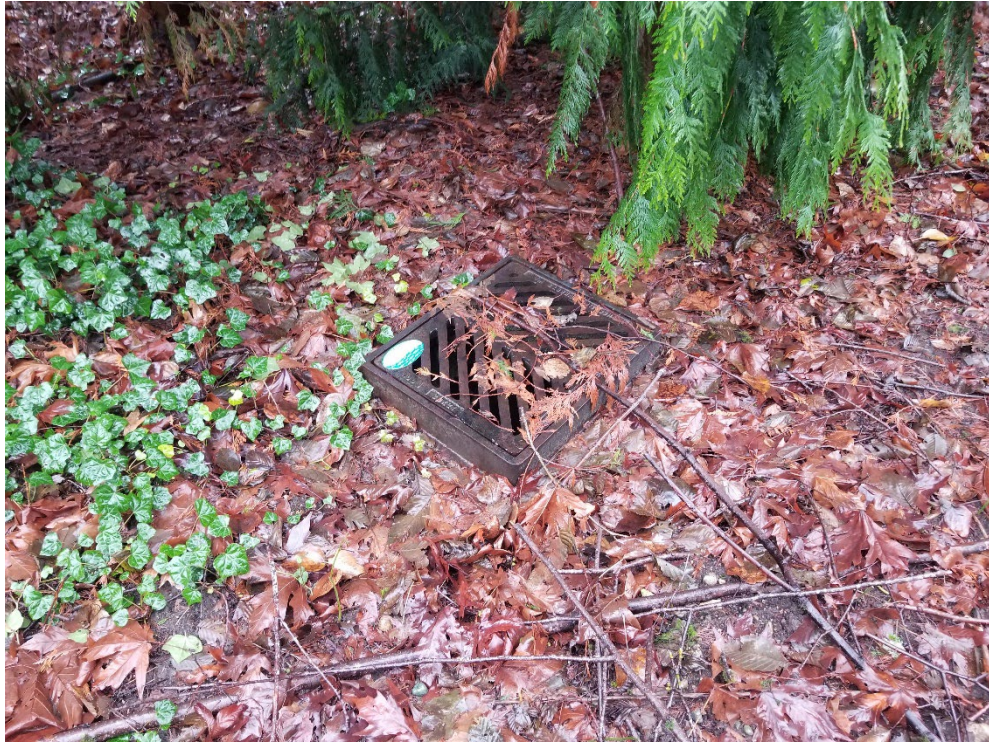
Photo 9—Catch basin inlet to the culvert that conveys the unnamed tributary near TP-1.
