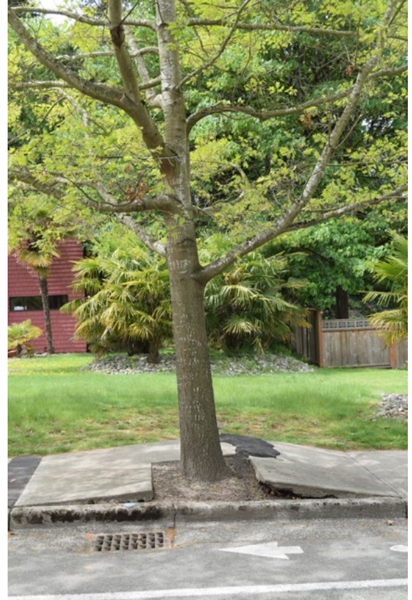
Heaved sidewalk on 112th Avenue NE is a tripping hazard
