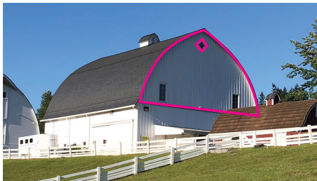
Kelsey Creek Farm barn roof shape and window
