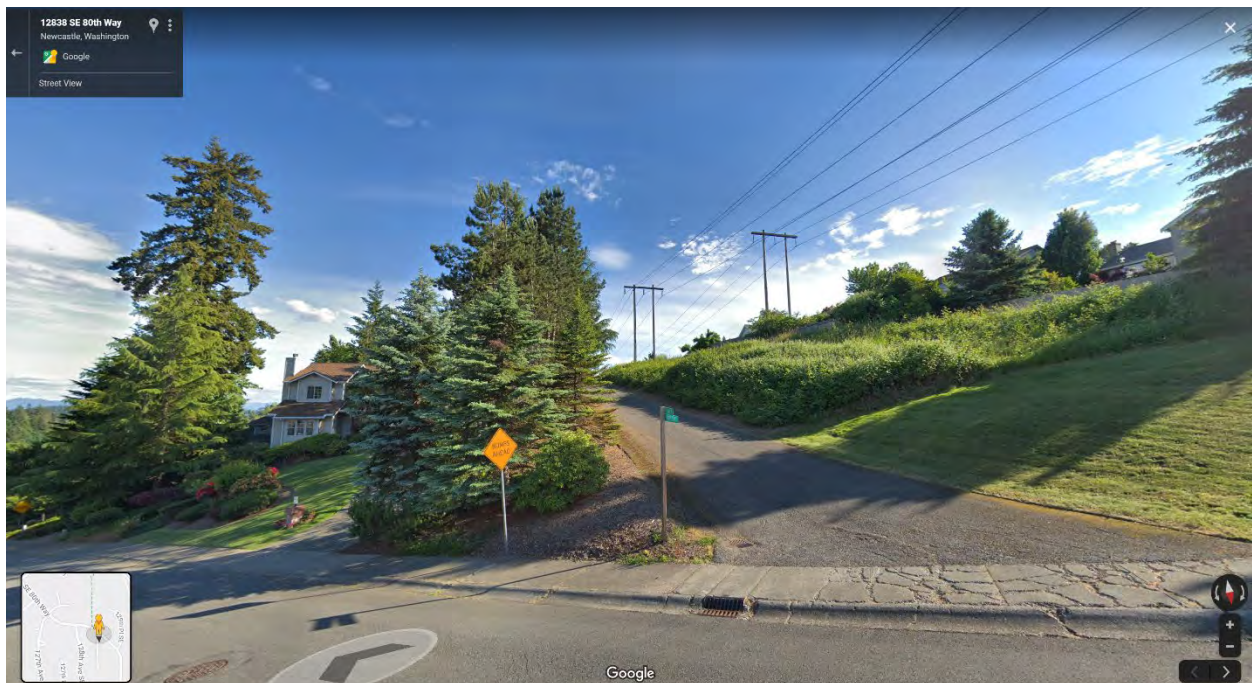
Figure 12. Current 115kV electric transmission facilities around 12828 SE 80th Way, Newcastle, WA 98056
