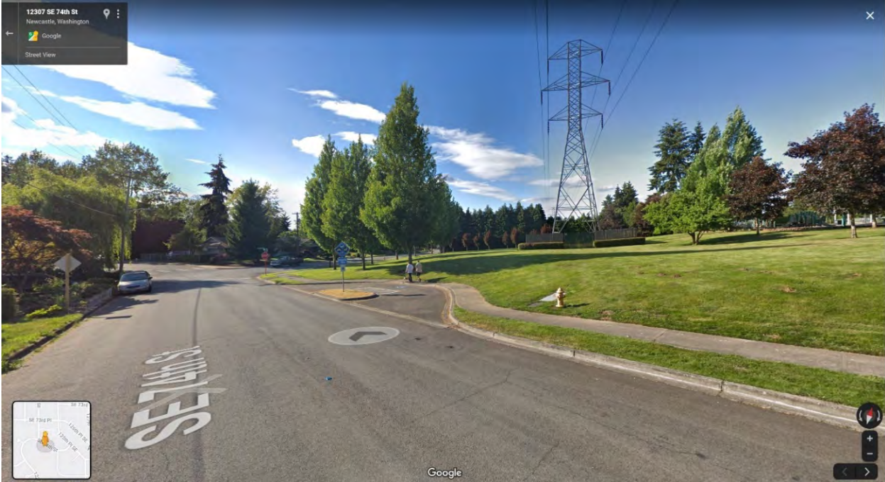
Figure 13. Seattle City Light 230kV Transmission Line at Donegal Park [SE 74th ST, Newcastle, WA 98056]
