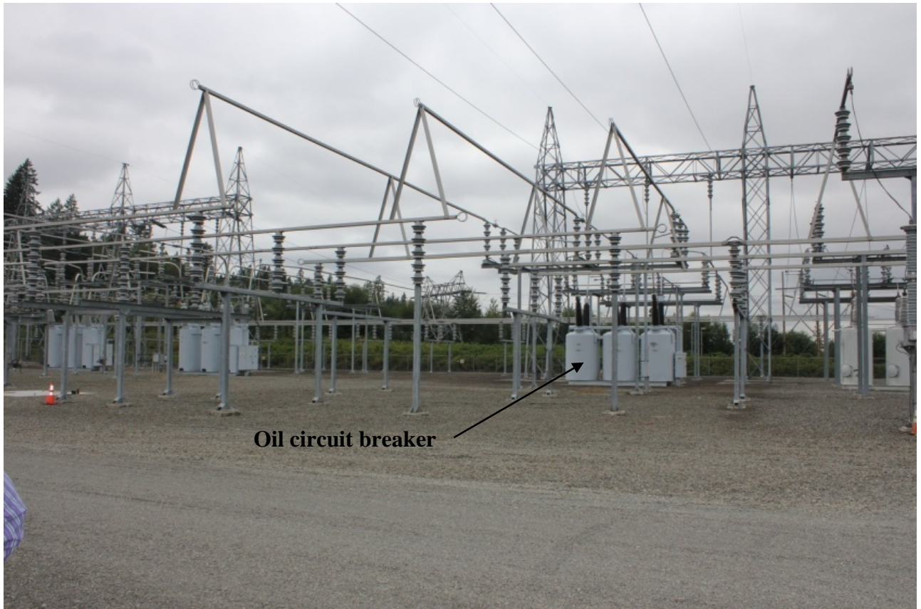
Figure 34. 230 kV Switchyard with Bulk Oil Breakers at Sammamish Substation
