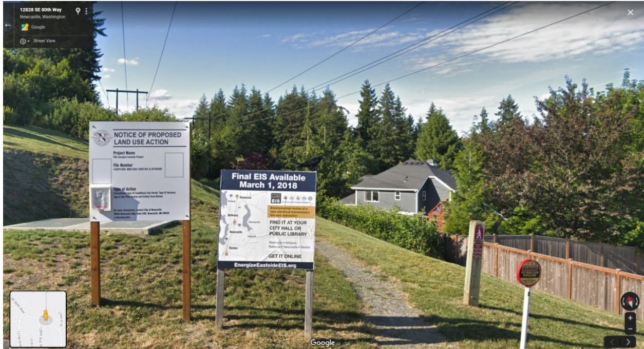
Figure 11. Existing two 115kV electric transmission facilities on H-frame poles travel in existing transmission corridor through Newcastle around SE 80th Way, Newcastle, WA 98056
