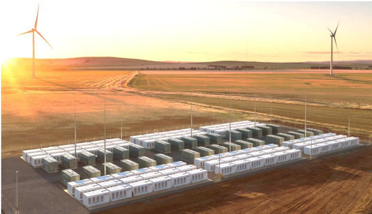
Figure 16: Hornsdale Power Reserve is 100MW/129MWh, approximately 43 times smaller than the Complete Solution 42
