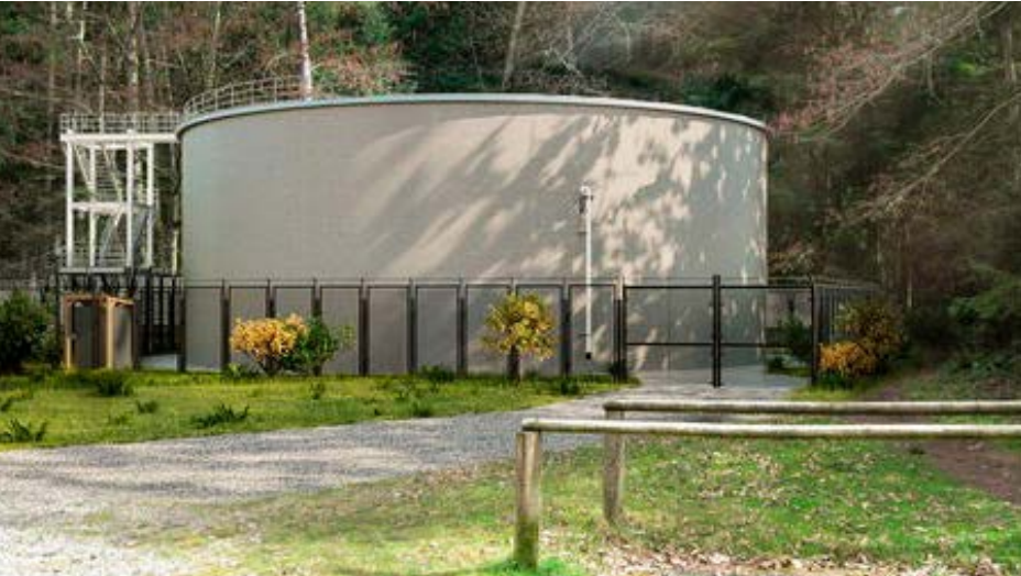
The new reservoir, shown in this visualization, will be made of concrete instead of steel.
