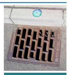
Stormwater flows off streets and sidewalks, enters storm drains and flows, without treatment, into streams, lakes, and wetlands.
