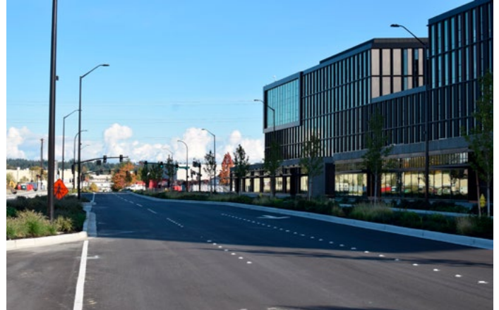
NE Spring Boulevard improvements between 120th and 124th avenues were completed in fall 2020
