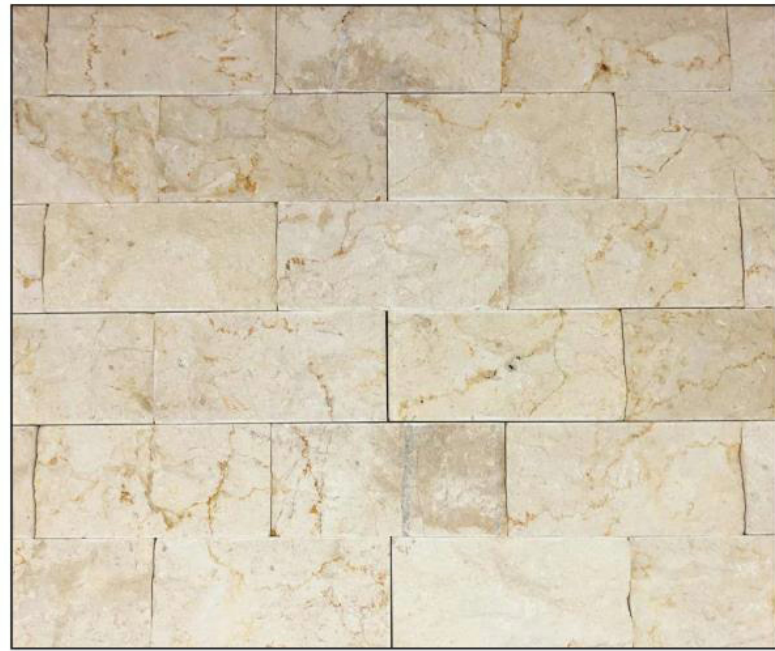
STONE VENEER AT GROUND STREET FACING FACADE
