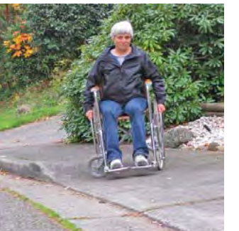
Steep driveway cross slope.
