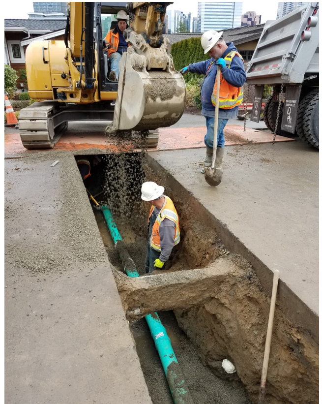
The Viewcrest Sanitary Sewer Replacement Project, completed in February of 2018, replaced over a half-mile of sewer pipeline. The improvements were performed as a scheduled upgrade of aging infrastructure.
