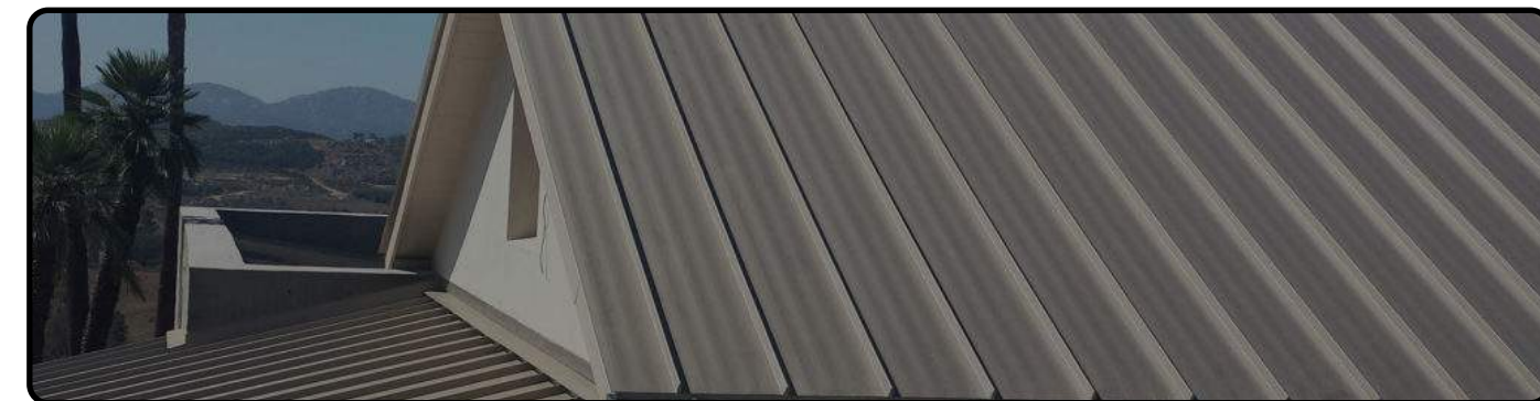
Standing Seam Metal Roofing
