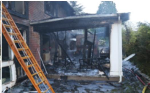
**May 24, 2018** – A barbecue left on overnight and installed closer to combustible materials than required by the manufacturer caused significant damage to the outdoor covered area and the interior of the residence.
