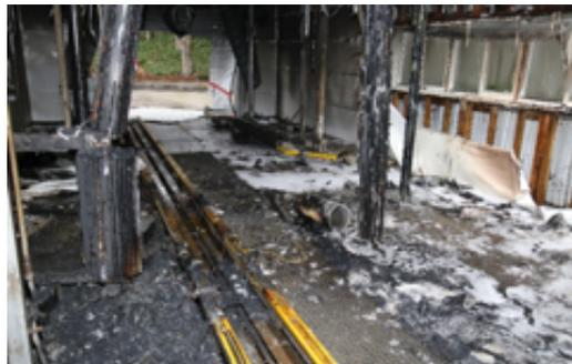
**December 10, 2018** – This car wash fire was caused by a heater too close to the soft foam car wash brushes. The heater had been used during a prolonged stretch of below freezing weather to keep the brushes from freezing.
