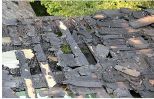
**August 9, 2018** – Spontaneous combustion of an oil-soaked rag used to stain a deck the previous day caused extensive damage to the roof of the attached dwelling.
