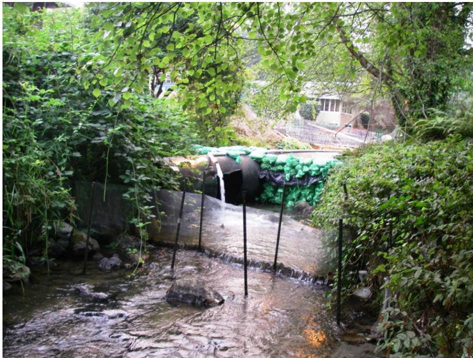
Figure 5-20. Construction weir blocking fish passage in Reach A, Coal Creek 6 September 2017.
