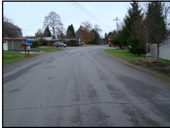
Northbound on 117th Ave SE South of SE 56th St
