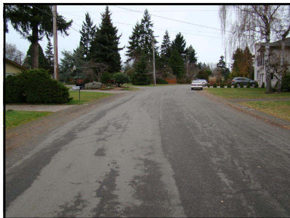
Northbound on 117th Ave SE South of SE 58th St
