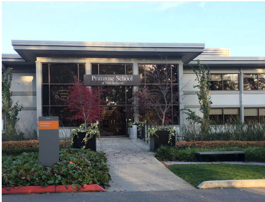
Photo 4. Zone 1 – Building monument (Primrose School)
