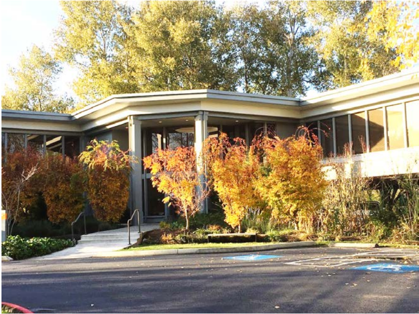
Photo 2. Zone 1 – Building entrance (Alderwood building)
