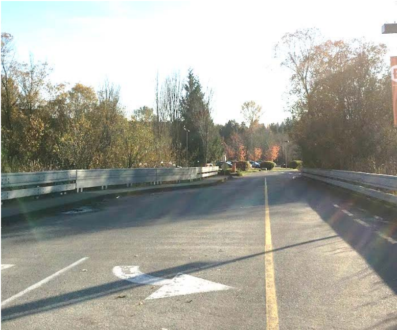
Photo 5. Zone 2 – Access road
