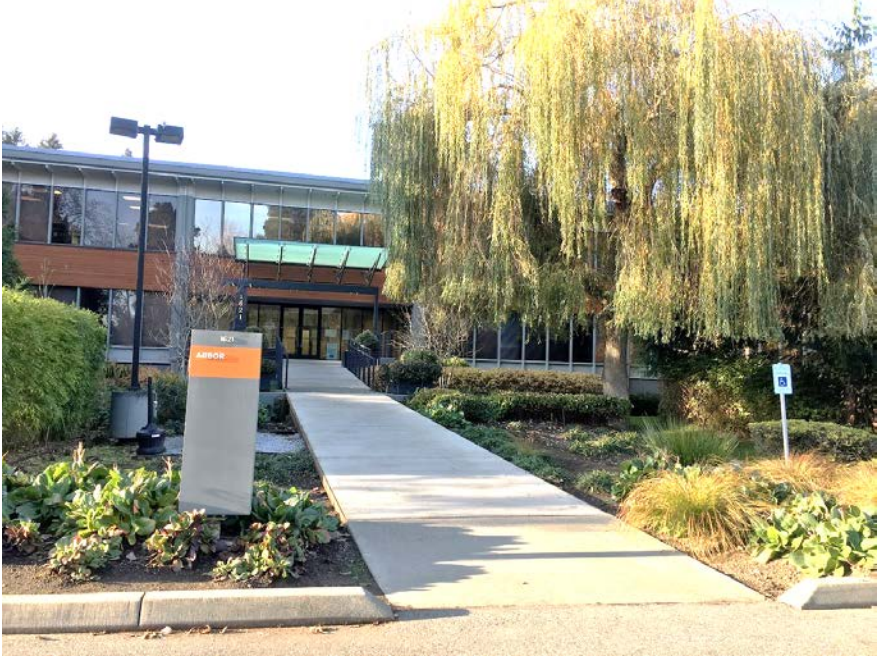
Photo 1. Zone 1 – Building entrance (Arbor building)
