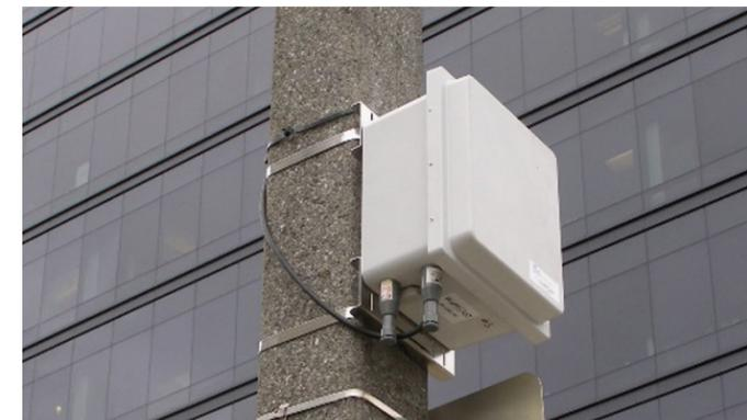
**Figure 24. BlueTOAD Travel Time Unit on a street light pole**
