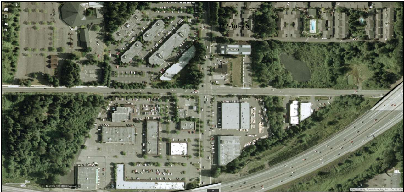
Evans Plaza buildings were built between 1968 and 1984. Image at 36 years old. (2002)
