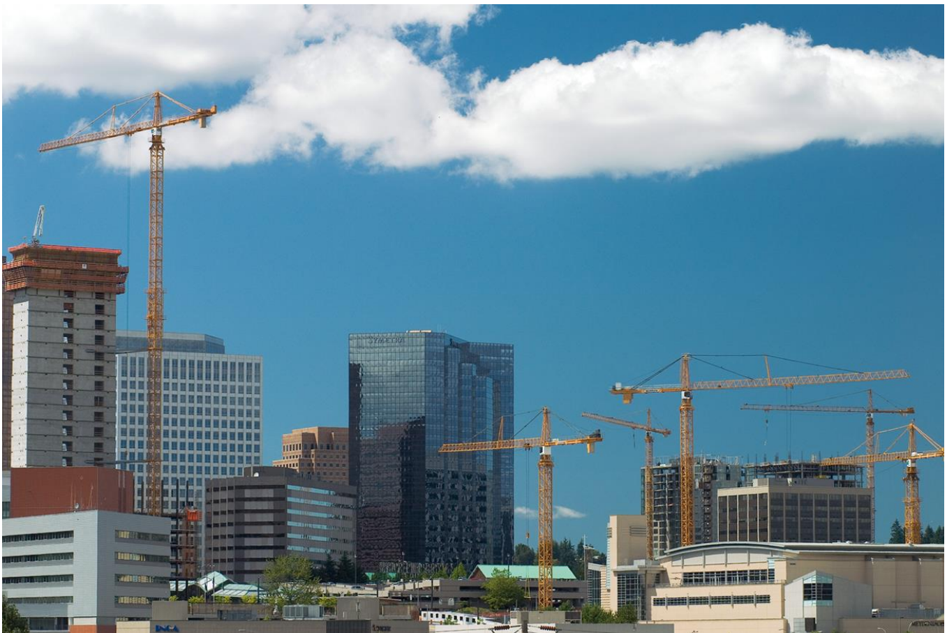
Construction cranes towering over high-rise buildings in Bellevue.
