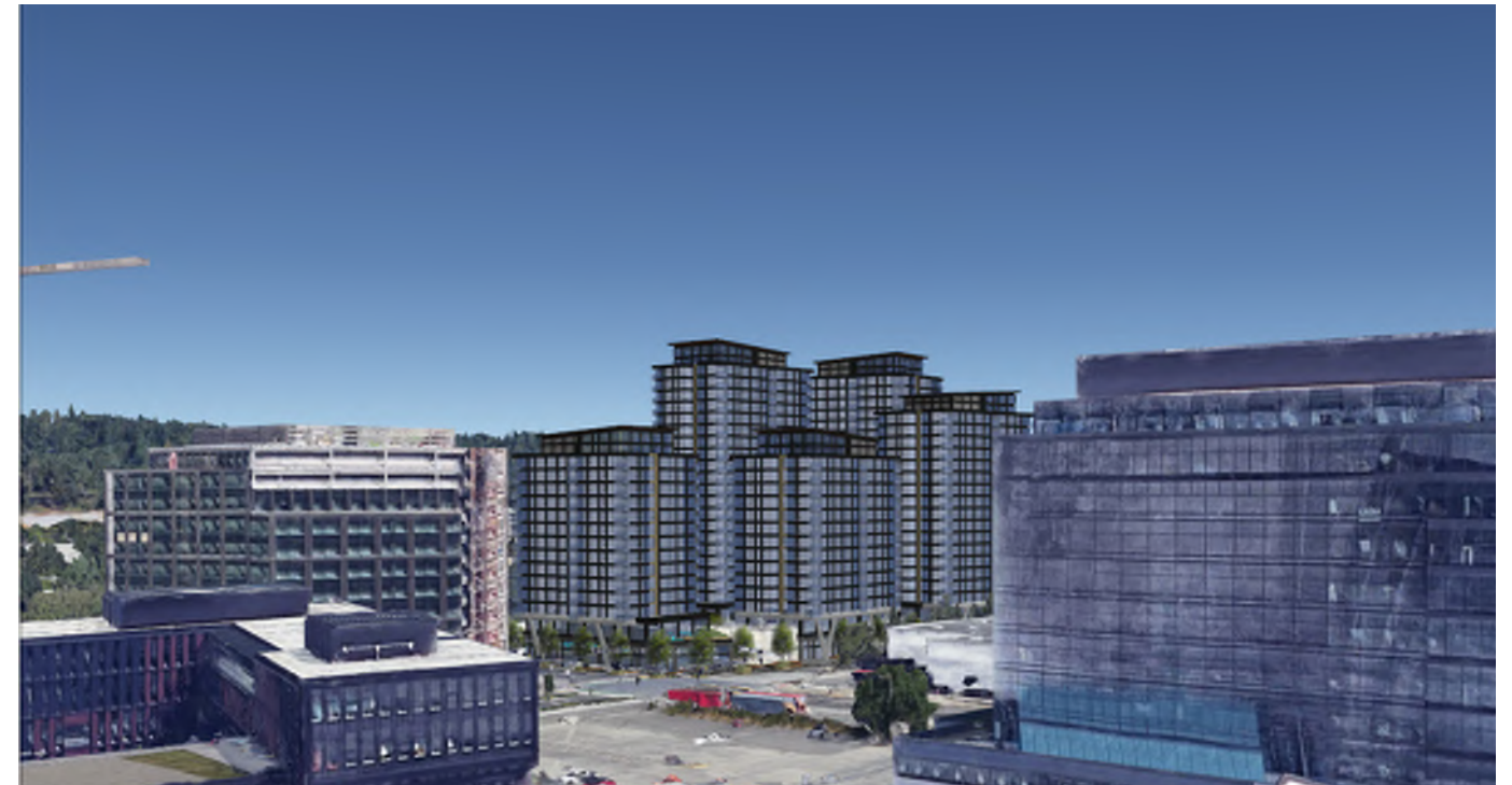
View looking NE
