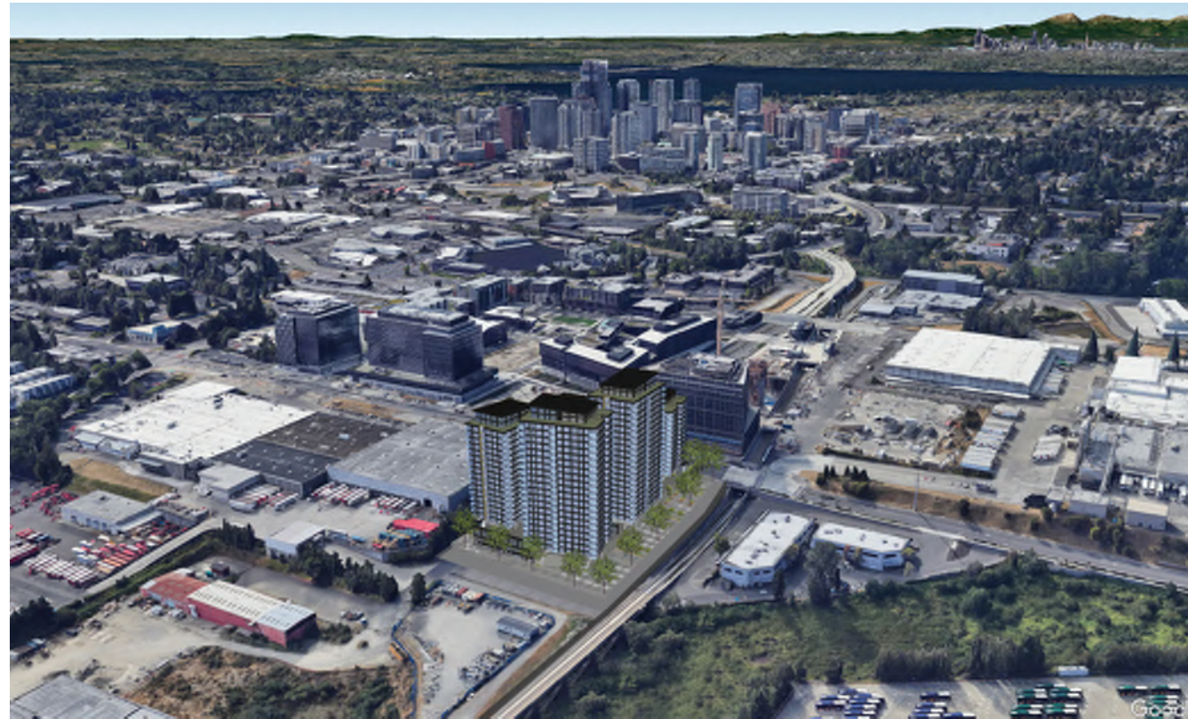
View looking SW
