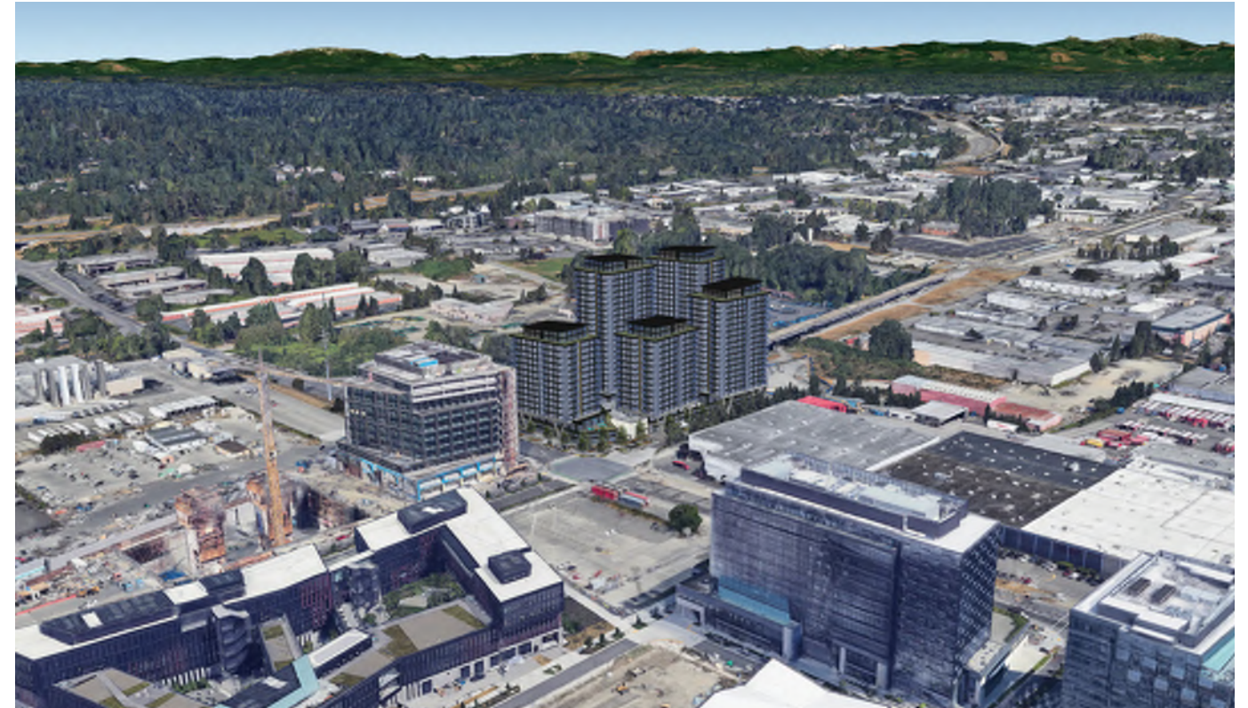
View looking NE
