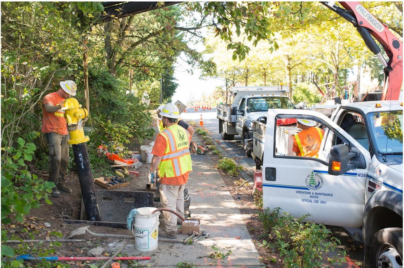
Bellevue Utilities workers repairing a fire hydrant on a street.
