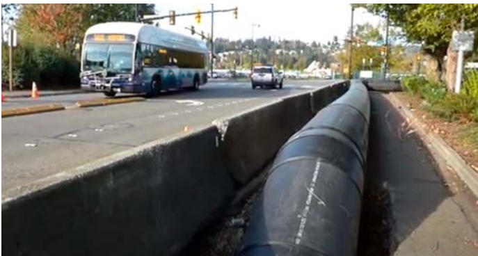
Example of a King County temporary detour pipe (Photo credit: King County)
