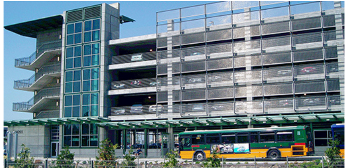
The Eastgate Park & Ride garage provides parking for transit users along I-90.
