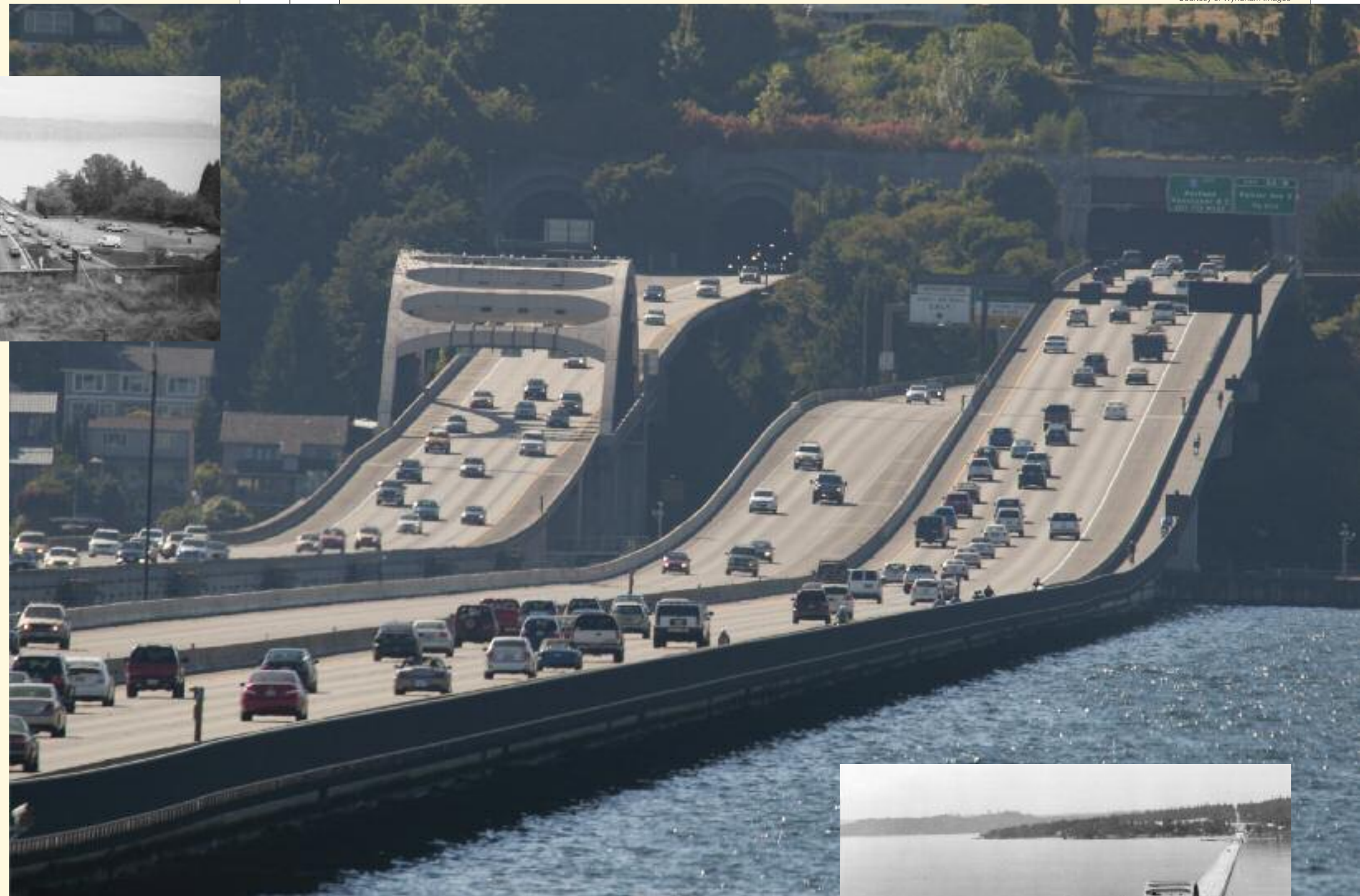
The spans today, as viewed from Mercer Island toward Seattle.
