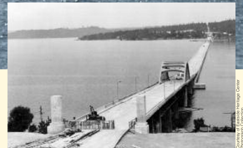
The "World Famous Pontoon Bridge" under construction approximately 1939 or 1940. The view is from Seattle east to Mercer Island.
