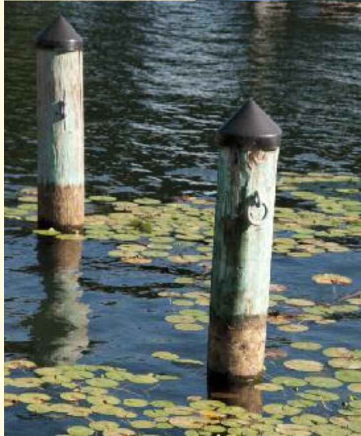
Pilings and lily pads at Bellevue Marina.
