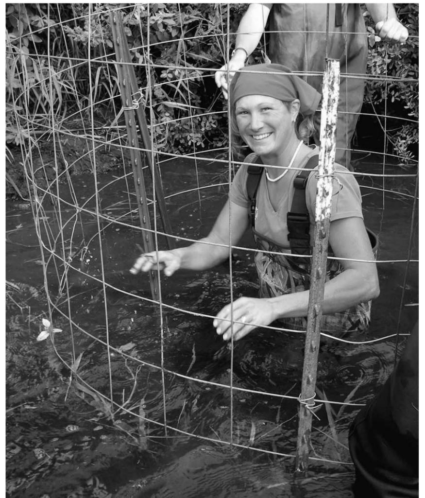
Utilities worker Trish Tyo helps install fencing around the opening of a pond leveller, placed in a beaver dam to allow salmon passage and stream flow.
