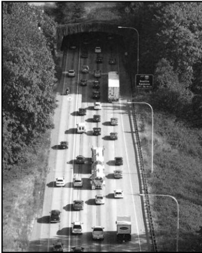
In 1972, the old State Route 405 was widened through Bellevue to create Interstate 405 and the Wilburton Tunnel was built. Now, 36 years later, it's time to widen the highway again and the tunnel must be removed to make room for two new southbound lanes.
