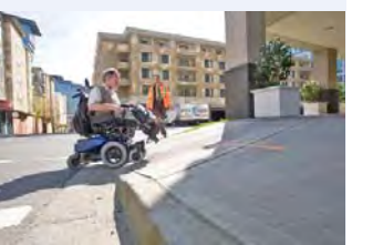
Steep ramp running slope.
