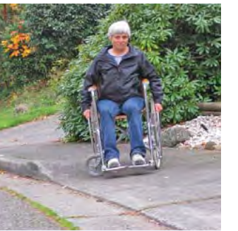
Steep driveway cross slope.
