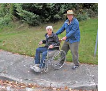
No ramp landing panel.
