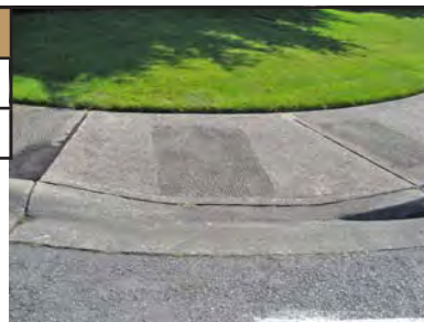
Non-standard detectable warning surface at SE 34th Street & 111th Avenue SE.
