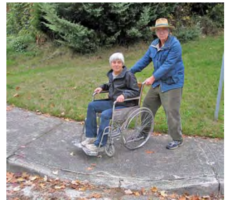
No ramp landing panel.
