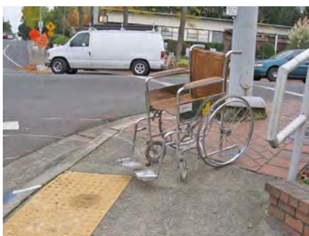
Steep ramp flare slope.
