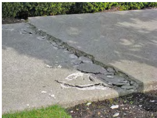
Two inch change in level in a concrete sidewalk at 58th Place & SE 58th Street.
