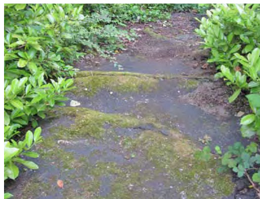
Change in level in an asphalt sidewalk at SE 27th Street & 124th Avenue SE.
