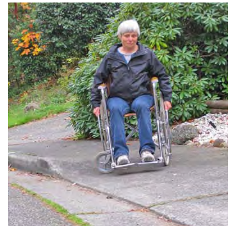
Steep driveway cross slope.
