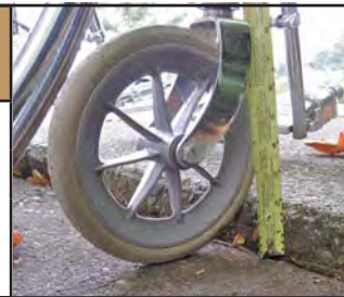
Change in sidewalk level (2 inch) at 148th Avenue NE & NE 35th Street.
