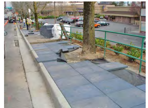
Rubber sidewalk panels at NE 10th Street west of 102nd Avenue NE allow tree roots to grow under the sidewalk without creating a change in level barrier for people with disabilities.
