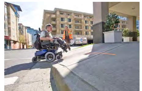
Steep ramp running slope.
