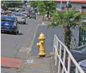
Hydrant on 3 foot sidewalk at Main Street & 107th Avenue NE renders sidewalk unusable to people with disabilities.
