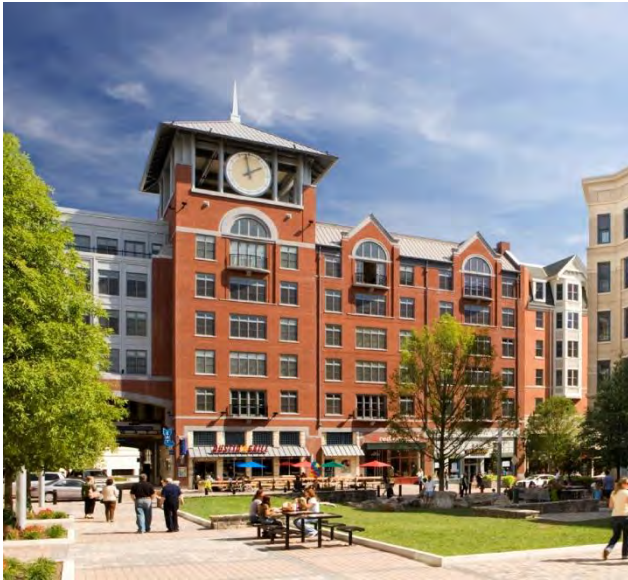
Identifiable Roof Forms
