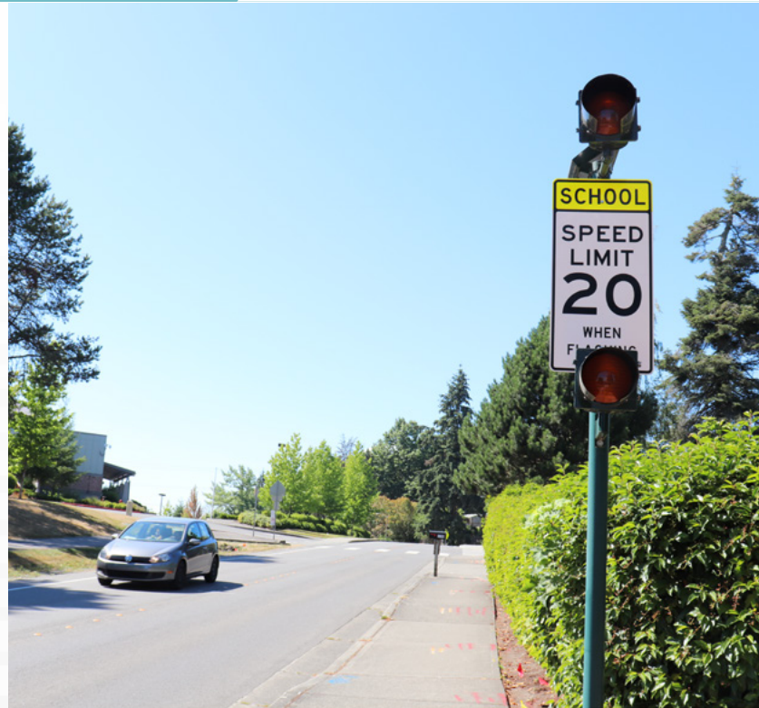
Figure 26. School zone flashing beacon near Woodridge Elementary School
