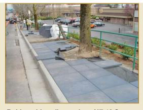
Rubber sidewalk panels at NE 10 St west of 102 Ave NE allow tree roots to grow under the sidewalk without creating a trip hazard.
