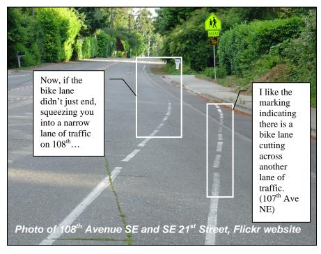
lanes on both sides of this corridor where not complete. This is accomplished with projects **B-138-E/W** which propose adding a 5 foot wide bike lane to both sides of 108<sup>th</sup> Avenue SE from Bellevue Way to SE 34<sup>th</sup> Street.
