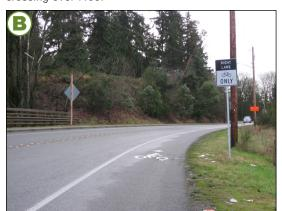
An 5 foot-wide bike lane runs along both sides of Lake Washington Boulevard SE from I405 to SE 60th Street, as well as an 8 foot sidewalk only on the east side.
