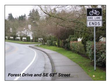
Between SE 63<sup>rd</sup> Street and 152<sup>nd</sup> Avenue SE Forest Drive consists of two travel lanes that occupy the 34 foot wide roadway for most of the corridor (several instances of center turn lanes). This corridor is envisioned as having bicycle lanes reflected in the new Pedestrian and Bicycle Plan which proposes project **B-158-N/S** which would add a 5 foot wide bike lane on the north side of Forest Drive SE from SE 63rd Street to Lakemont Boulevard SE..
