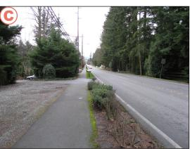
Looking nouth, the recently constructed 6 foot-wide porous asphalt pathway and planter strip/buffer can be seen on the west side.
