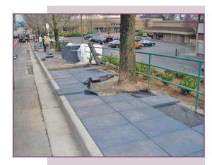
Rubber sidewalk panels — made of recycled tires — at NE 10th St west of 102nd Ave NE allow tree roots to grow under the sidewalk without creating a trip hazard.
