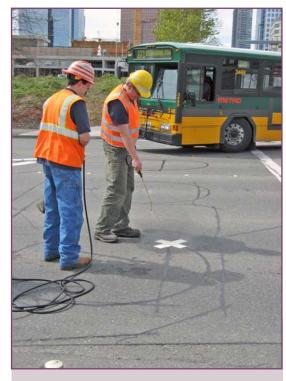
Bellevue staff applying the torch-down "x" marking the location of a bicycle actuated signal.
